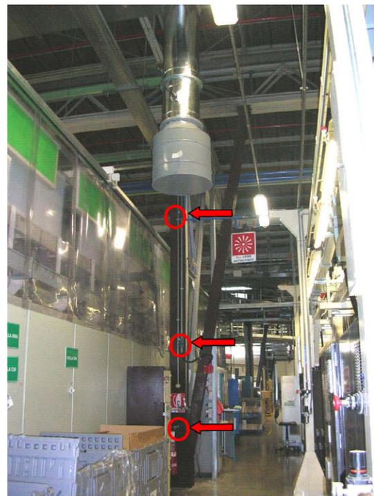
Fig. 11. Temperature sensors location and RHDVS test diffuser.
