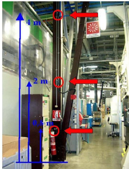
**Fig. 8.** Temperature sensors location.
