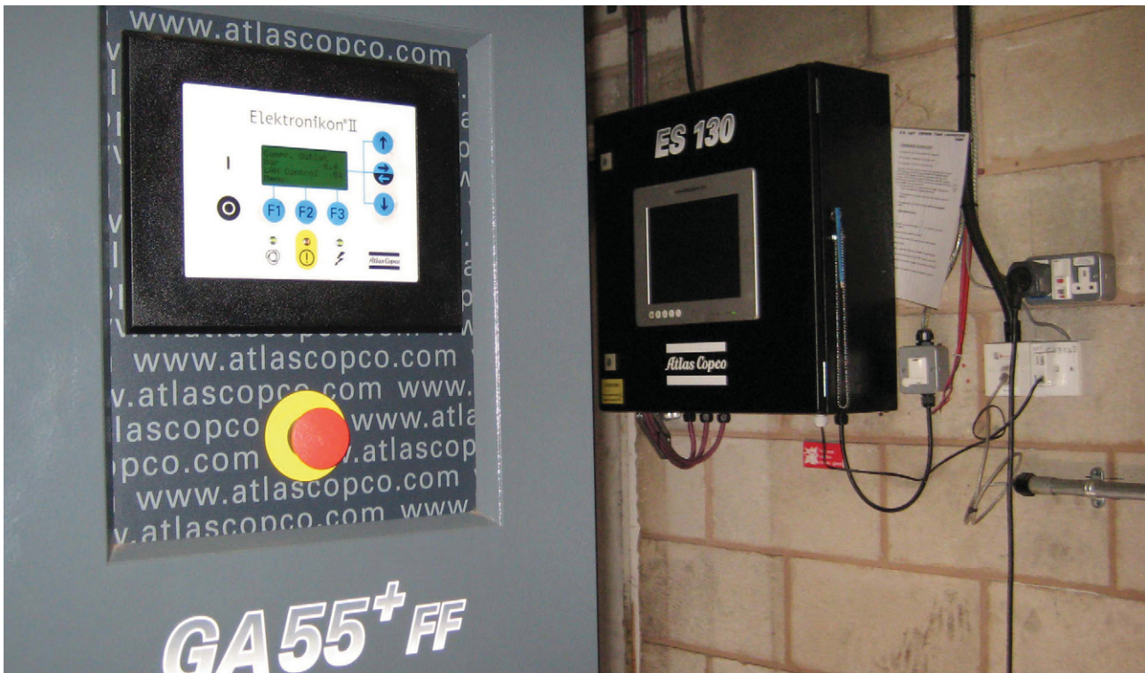
Figure 2. Atlas Copco's AIRScan audit team recommended the ES 130 unit to control output and the AIRConnect for remote monitoring.
