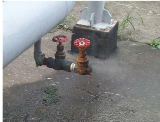
b. leaks at open valve to drain water
