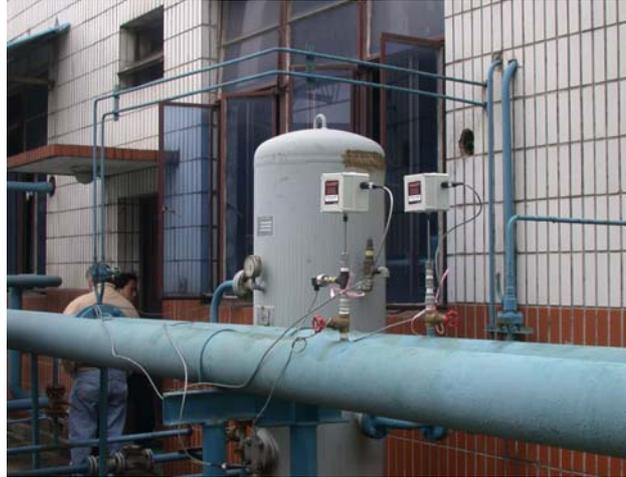
**Figure 2 flow measurement with insertion-type mass flow meter**
