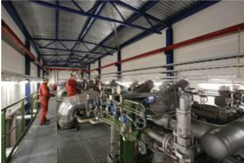
Fig. 5. CO<sub>2</sub> recovery with PSA system at a Finland refinery hydrogen plant (valve skid)
