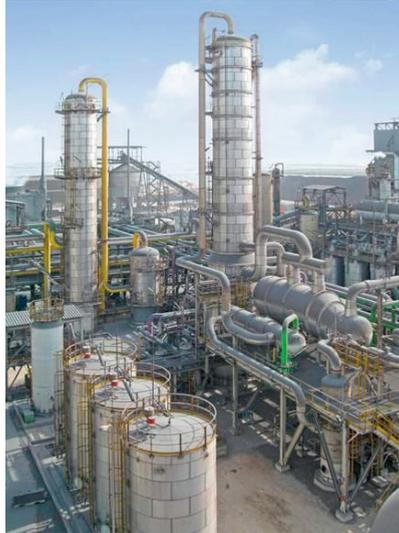
Fig. 9. CO<sub>2</sub> Absorption Unit in a DRI plant.
